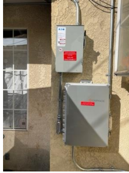
Installed Inverter
